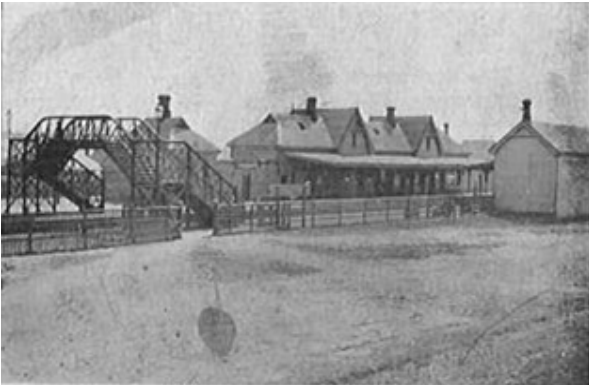
Sydenham Railway Station (1910)
