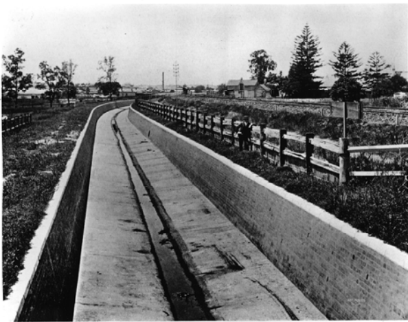
Marrickville Stormwater Drainage Channel (1899)
